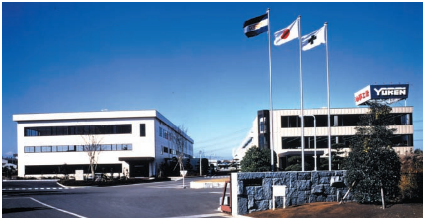
● Sagami Plant Front Gate
